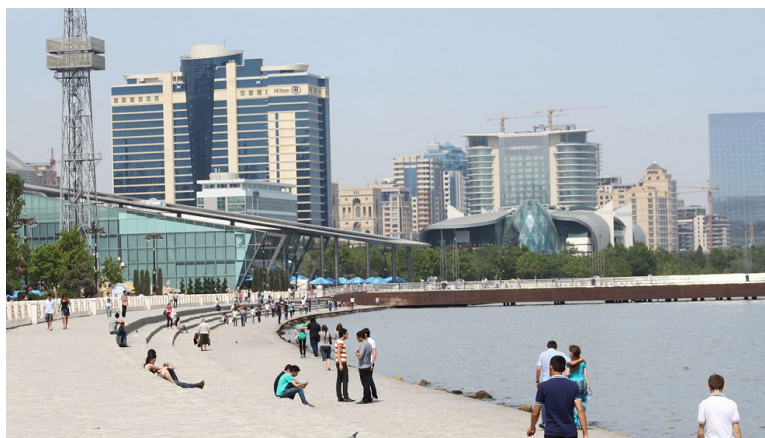
Tiered embankment adapted to fluctuations in the Caspian Sea level
