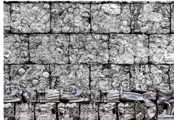
Detail of the recycled compressed aluminium blocks facade
