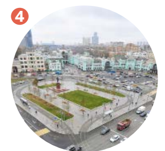
4 Reconstruction of the square and the railway station «Astrakhan - 1»
